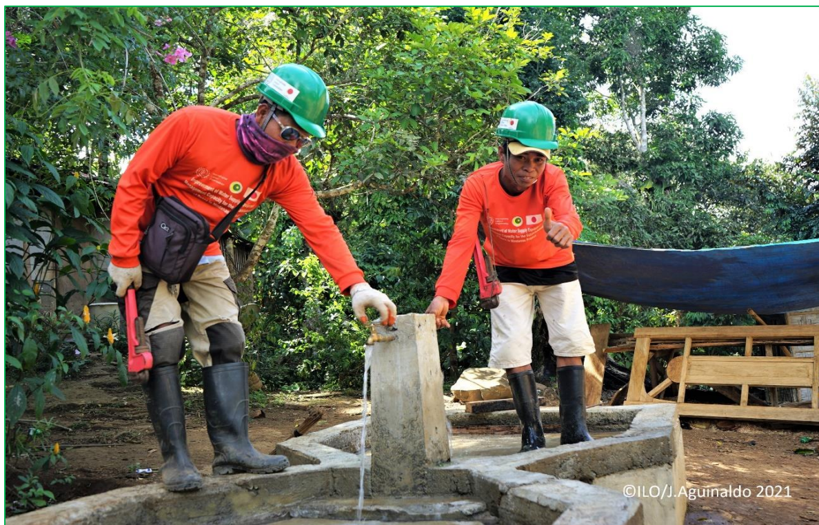
Test run in one of the tap stands in Looy, South Upi.
